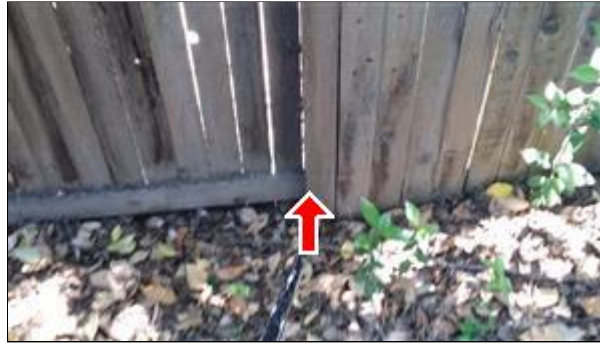
2.6 Picture 5 Rotted Fence Post (Left Side)
