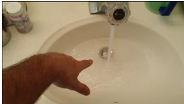
6.1 Picture 7 Slow Drain (Right Sink Master Bathroom))
