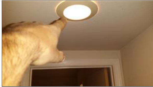
7.2 Picture 5 Flickering Light (Hallway)
