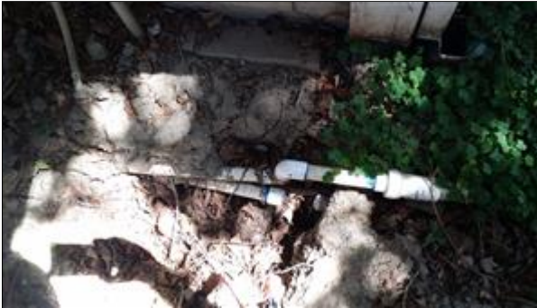
6.1 Picture 2 Exposed Plumbing (Right Rear)
