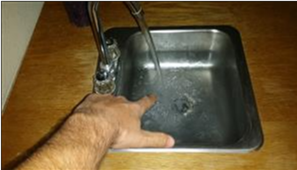
6.1 Picture 3 Slow Drain (Wet Bar)
