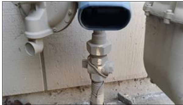
6.5 Picture 2 Close Up
