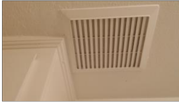
9.2 Picture 1 Dirty (Laundry Room)
